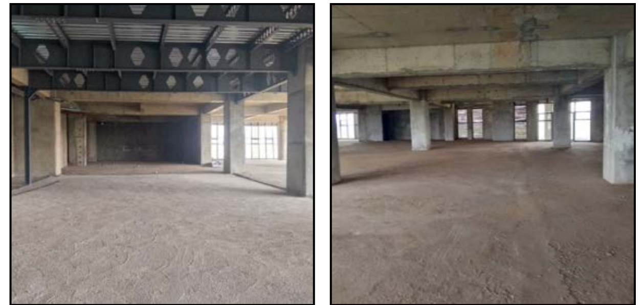
Internal Views of the Grey Boxes in the Tower
